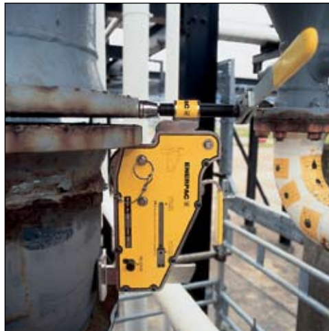
▲ Enerpac 3PCU8 flange alignment tool used to align a large flange
