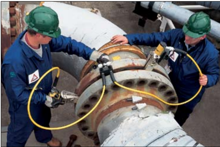
▲ Two 4PU56 Hydraulic Flange Spreaders used simultaneously to separate a flange
